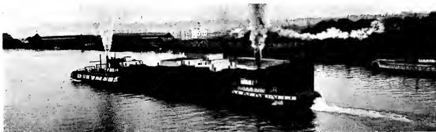
The "Vesterlide" being towed to the plant of the Willamette Iron and Steel Works to receive her boilers.
